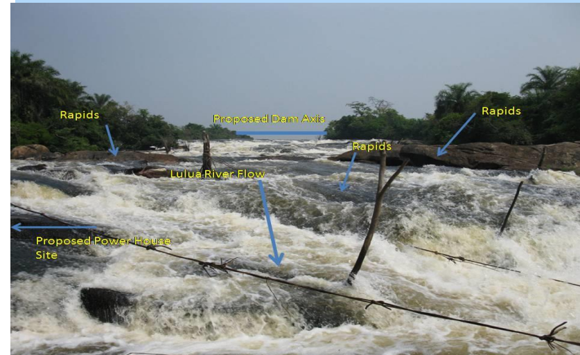
View of the River at Site of Katende H.E. Project
