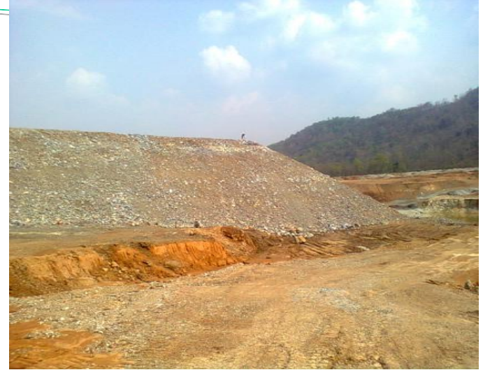
Stung Tasal Dam Site – work in progress
