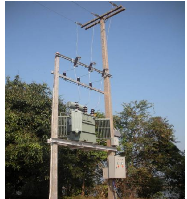
Installation of 22 kV electric network at Strung Trung to Kratie
