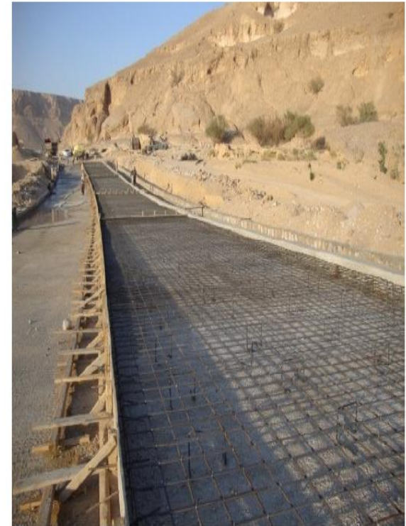
Slab Construction of Irish Crossing at Al-Ghurf Sah Road, Yemen
